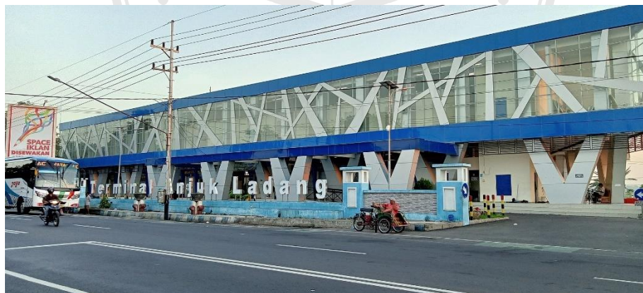
Gambar 2. 12 Tampak Terminal anjuk landing
