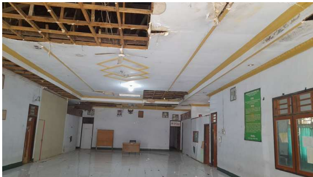
Lampiran. 3 Eksisting Interior Aula
